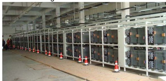
5 MW/10 MWh VRB - Rongke Power - China
